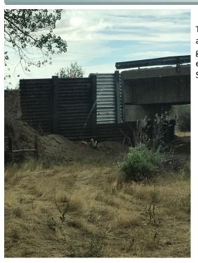
Photo and Update by Wayne Harris The bridge abutments have been fixed and approaches at both end of bridge have been graded. They will asphalt 50' to 100' on each end of the bridge. Heavy work is completed. Stay tuned and check crci.org for updates.
