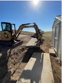
On June 13 a mini excavator was delivered onsite, and we started preparation for the 10' wide subgrade expansion of the concrete firing line on the High Power (HP) 1000-yard line. Several slabs of the existing sidewalk were removed and relocated to the existing HP sheds. Final grading of the subgrade was completed for the 8' wide expansion of the concrete firing line. Subgrade was also graded for the new 4' wide sidewalk from the parking lot to the existing crosswalk.
