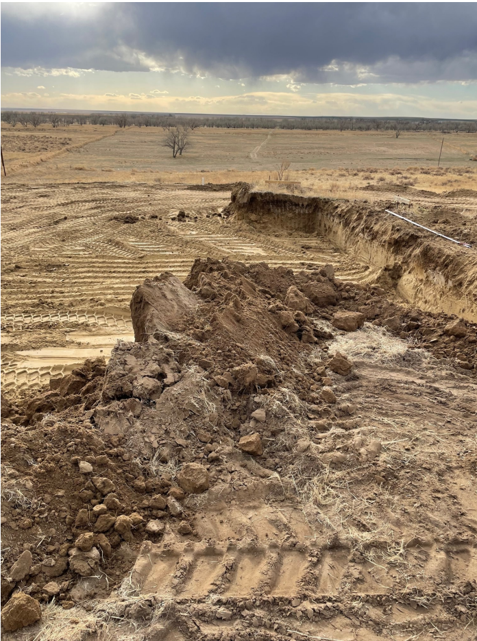
Early earthwork - Photo by Wayne Harris
