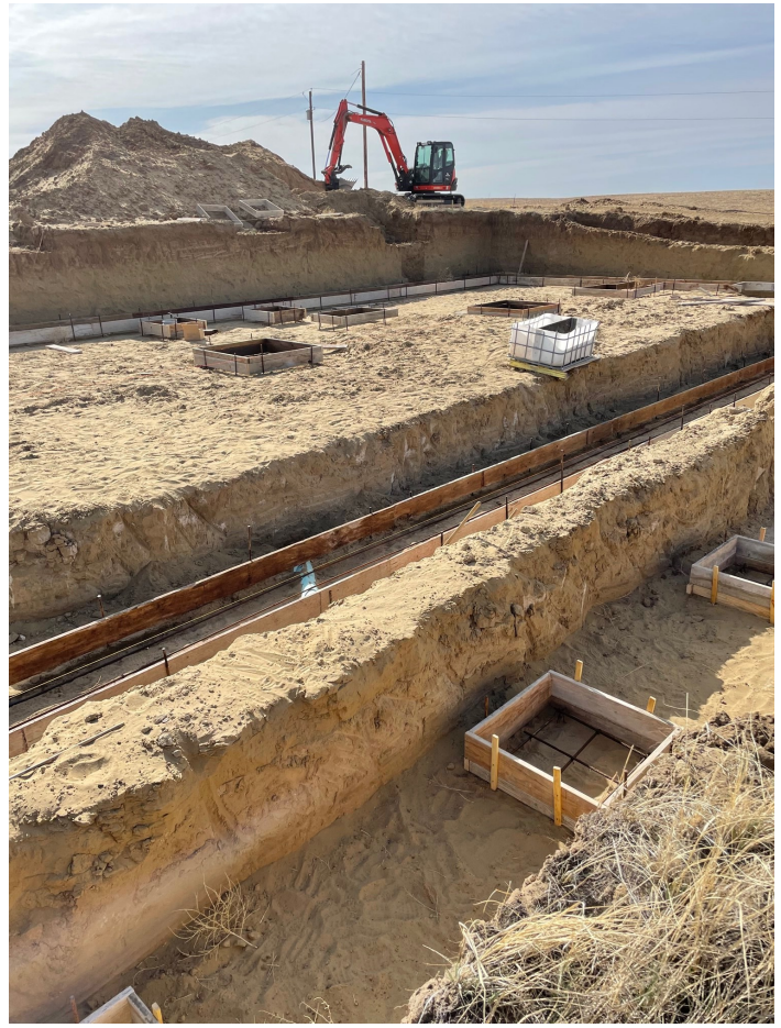
Clubhouse foundation - Photo by Wayne Harris
